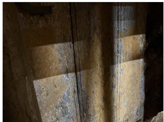
GF, T&G bead-butt boarding in the stabling to RTH
